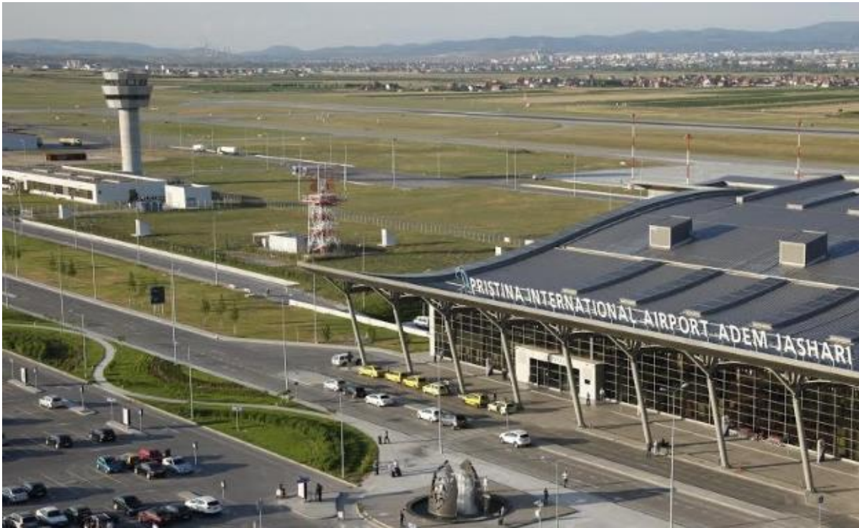
Figure 10. ATC tower, the premises of ANSA and PIA “Adem Jashari”
