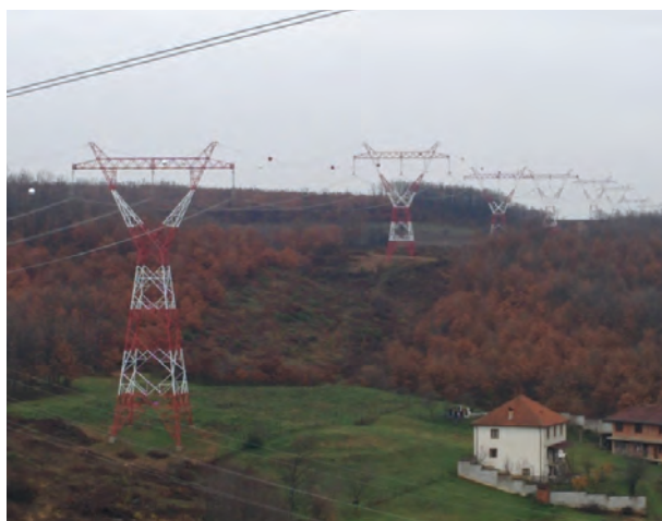
High-voltage transmission line markings
