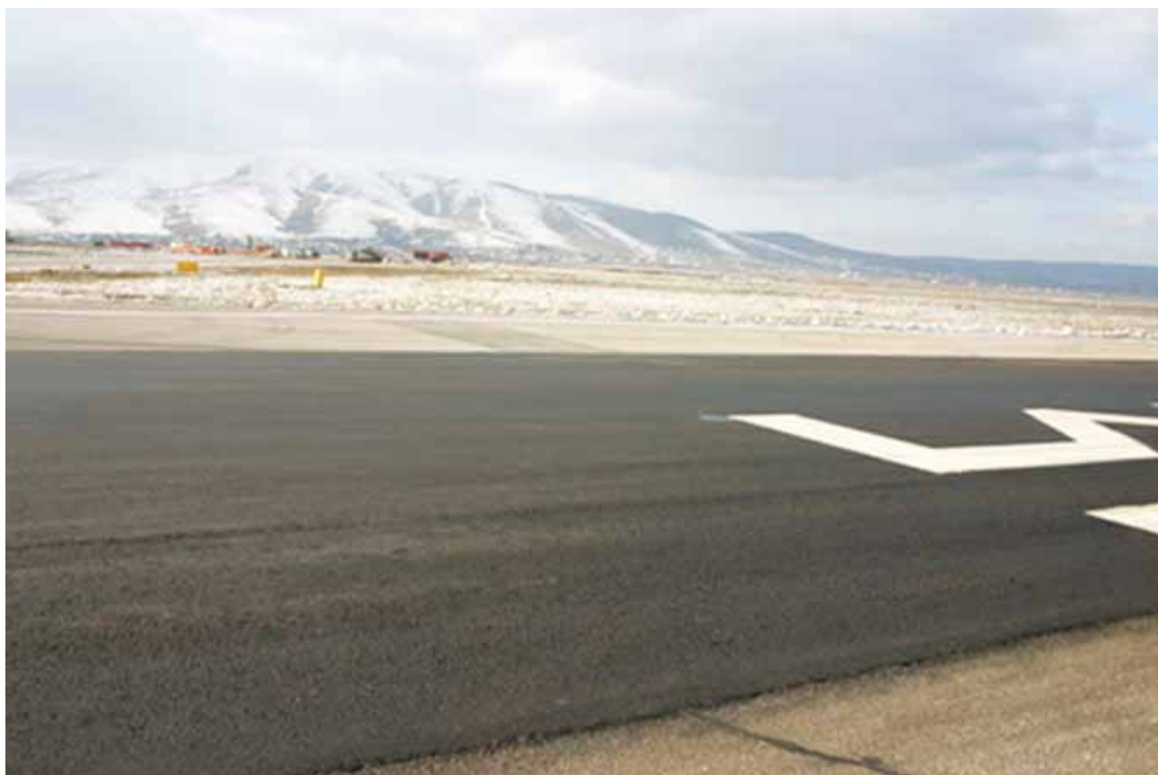
Resurfacing of the Runway at Prishtina International Airport "Adem Jashari"
