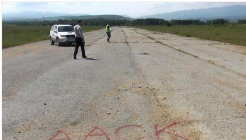
Photo 20 - Images from airfield in Ferizaj upon CAA inspection visit
